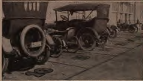
By Numbering the Parking Spaces about a Naval Reservation, the Various Motor Vehicles are Easily Found
